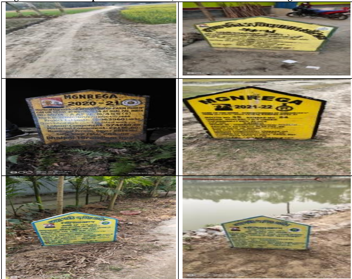
Figure 1.5: Assets inspected in Gobra Chhara, Dhalpal-I, and Chowdhurihat GPs
