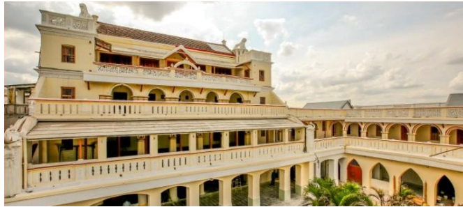
Fig. 9: Muktyala Palace, Krishna District, Andhra Pradesh- Repaired and Restored by the Family (Picture and Project by GSV Suryanarayana Murthy, Kshetra Consultants)
