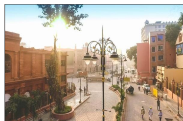
Pic. 1: Segregated pedestrian, vehicular movement
