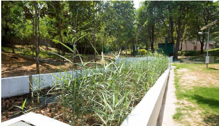
Fig. 2: Phragmites used for treatment of sewage water
