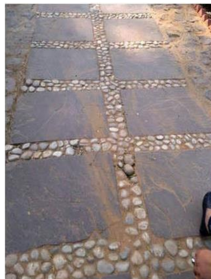
Fig. 9: Pebbles used in pathways to retain rainwater
